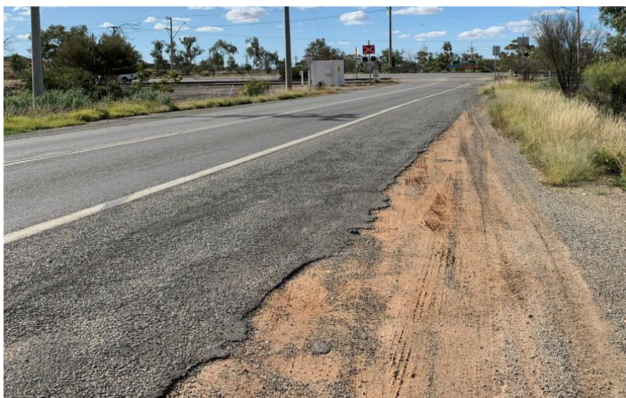
Figure 24: Entrance 1 sight distance (north-east)
