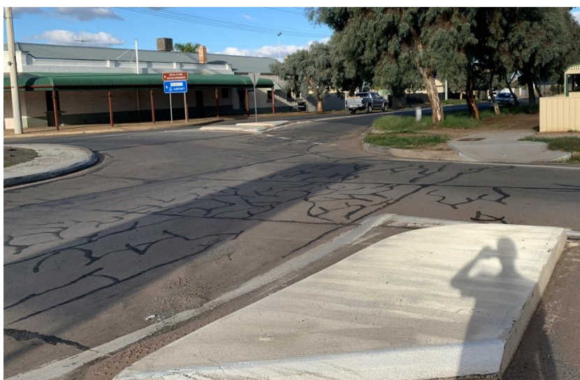
Figure 18: Sight distance (south-western approach, looking south-east)
