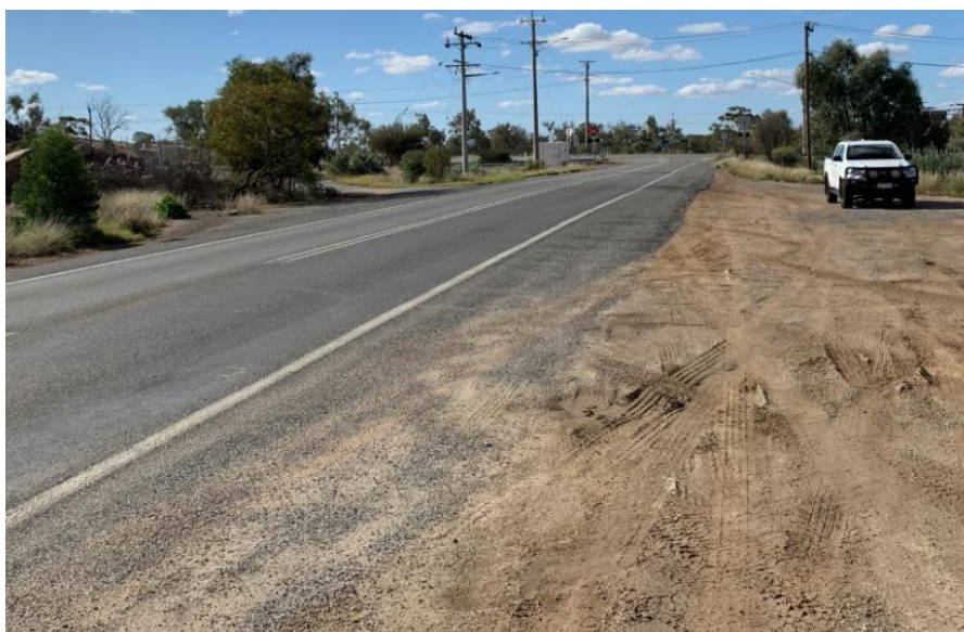
Figure 26: Entrance 2 sight distance (north-east)
