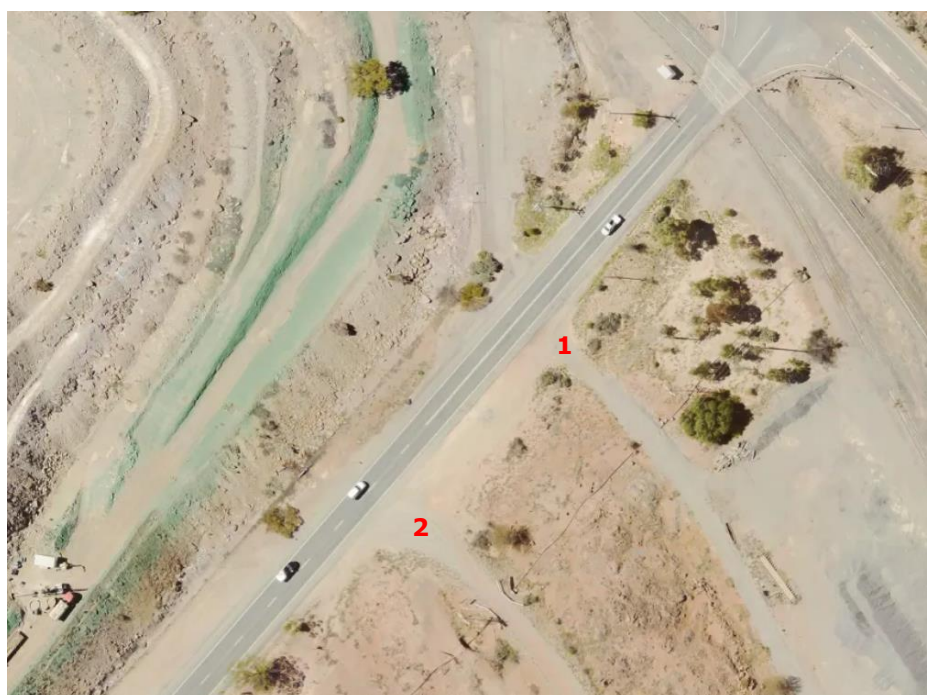
Figure 23: Existing Rail Facility entrances off Holten Drive
