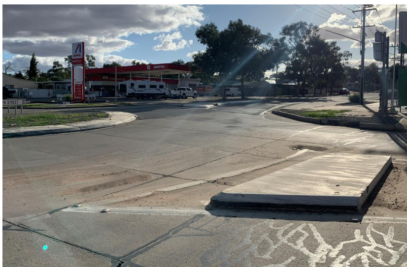
Figure 17: Sight distance (north-eastern approach, looking north-west)
