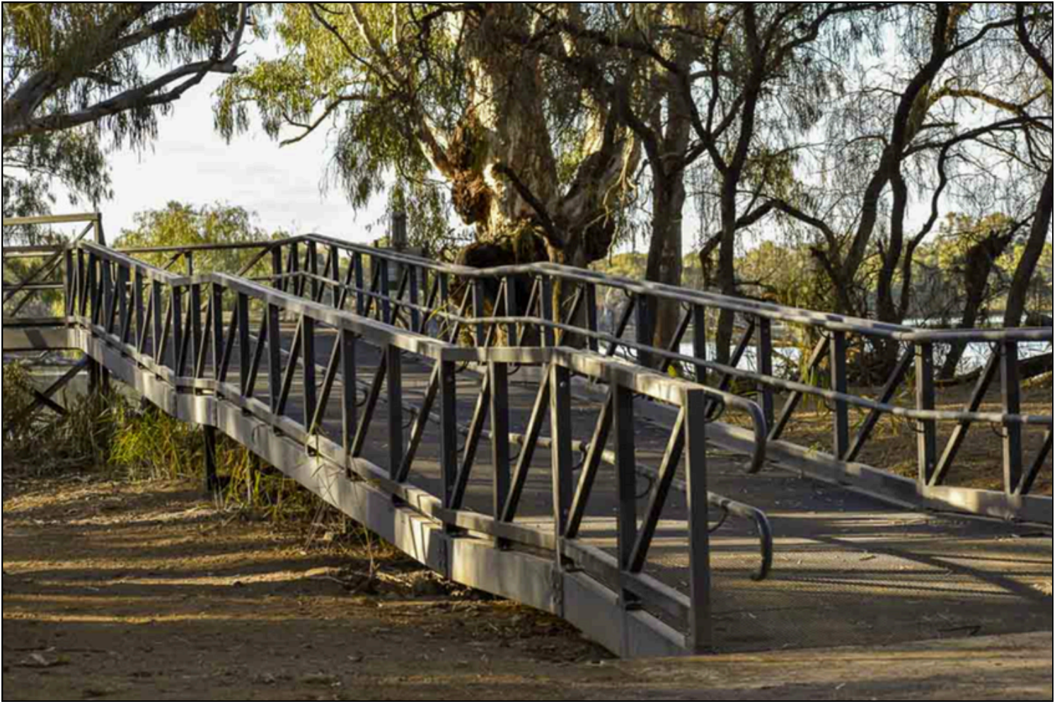
The completed Junction Island Bridge.
