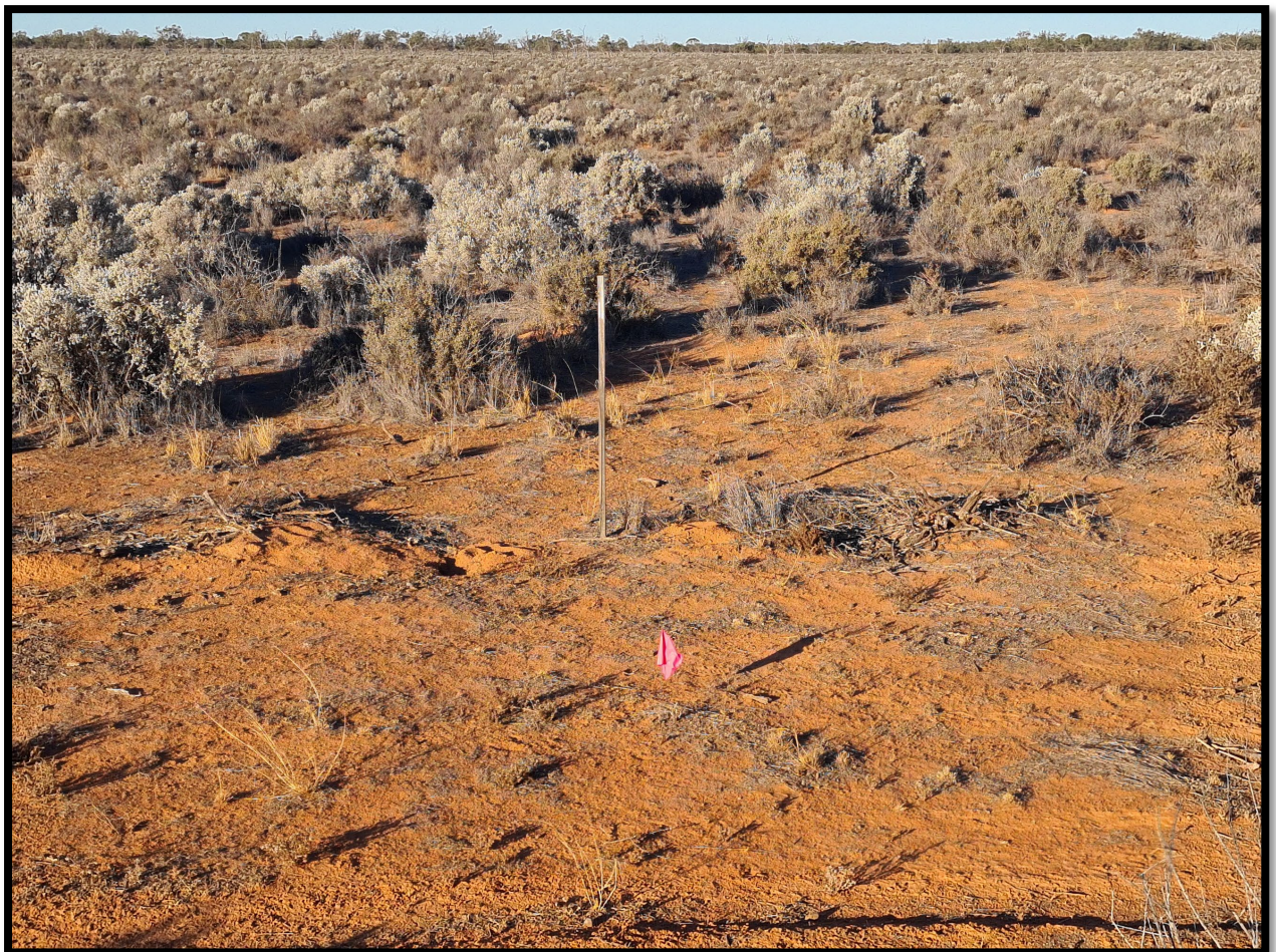
Plate 1: Pre excavation of drill pad
