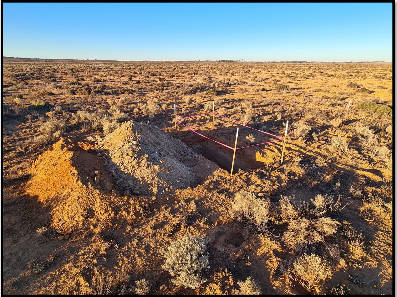
Plate 2: Drill pad with separated and stockpiled soil from spoil pit, before borehole drilling.
