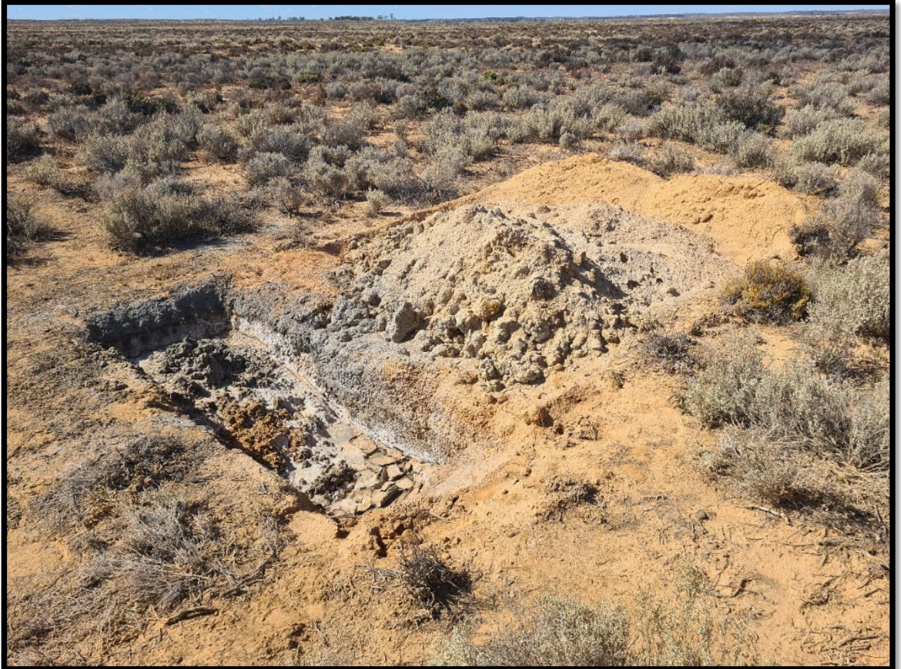
Plate 3: Post excavation and bore construction - spoil in pit and separation of topsoil and subsoil
