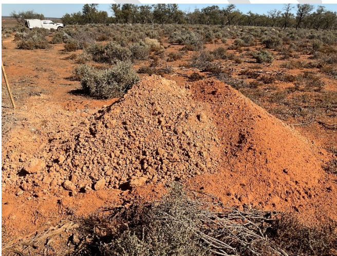
Figure 5 Topsoil and subsoil stockpiled beside sump
